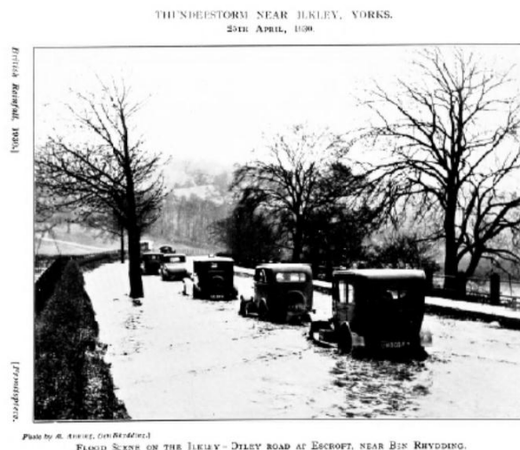
Photo G.1: Flooding at Escroft, just west of Burley in Wharfedale
